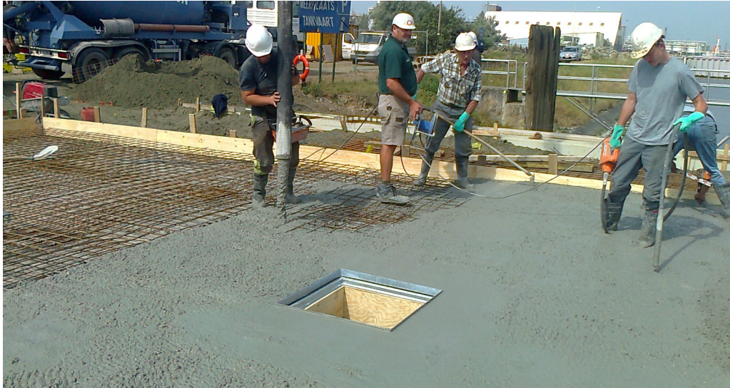
EE2 flooring concrete (30 M% replacement of the coarse fraction with recycled concrete aggregates) in case study 5 (Port of Antwerp)
