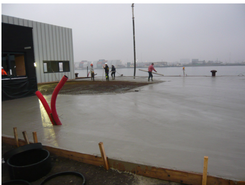
EE3 flooring concrete with recycled concrete aggregates in case study 5 (Port of Antwerp)
