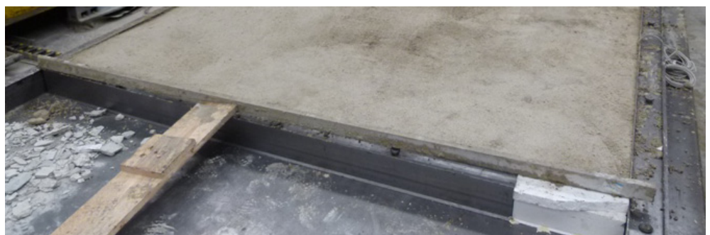
EE3 flooring concrete with recycled concrete aggregates in case study 5 (Port of Antwerp)
